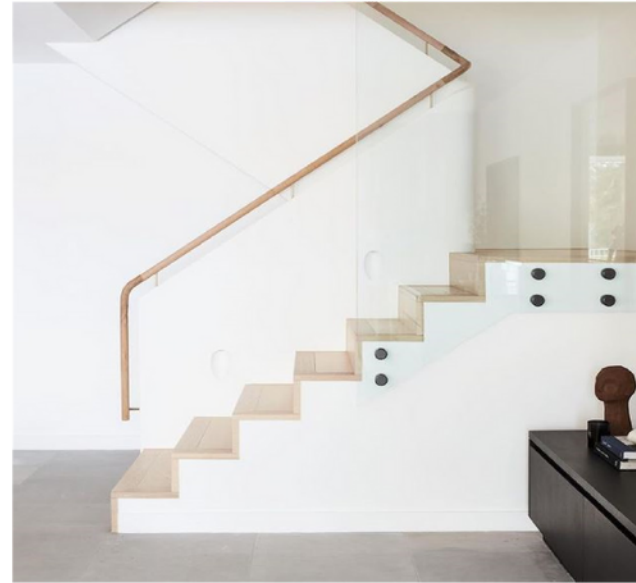
LOW LEVEL PLASTER LIGHTS INSTALLED FOR PATHWAY LIGHTING AT NIGHT
