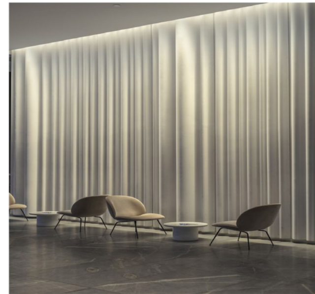
FLEXIBLE LED INSTALLED IN PELMET TO WASH DOWN ONTO CURTAINS
