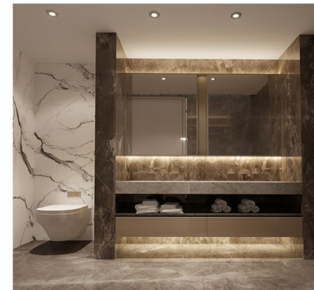
LED INSTALLED UNDER BATHROOM VANITIES TO CREATE A FLOAT EFFECT
