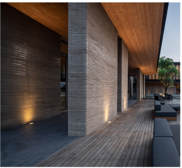
PIN LIGHTS INSTALLED AS INGROUND UPLIGHTS TO WASH UP AND HIGHLIGHT FEATURE STONE WALLS
