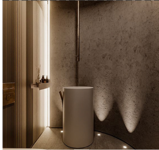
COLOUR CHANGING DOWNLIGHT INSTALLED TO SOFTLY HIGHLIGHT CEILING SURFACE MOUNTED SPOUT AND CCT LED INSTALLED IN CEILING TO SOFTLY FRONTLIGHT FEATURE TEXTURED WALL
